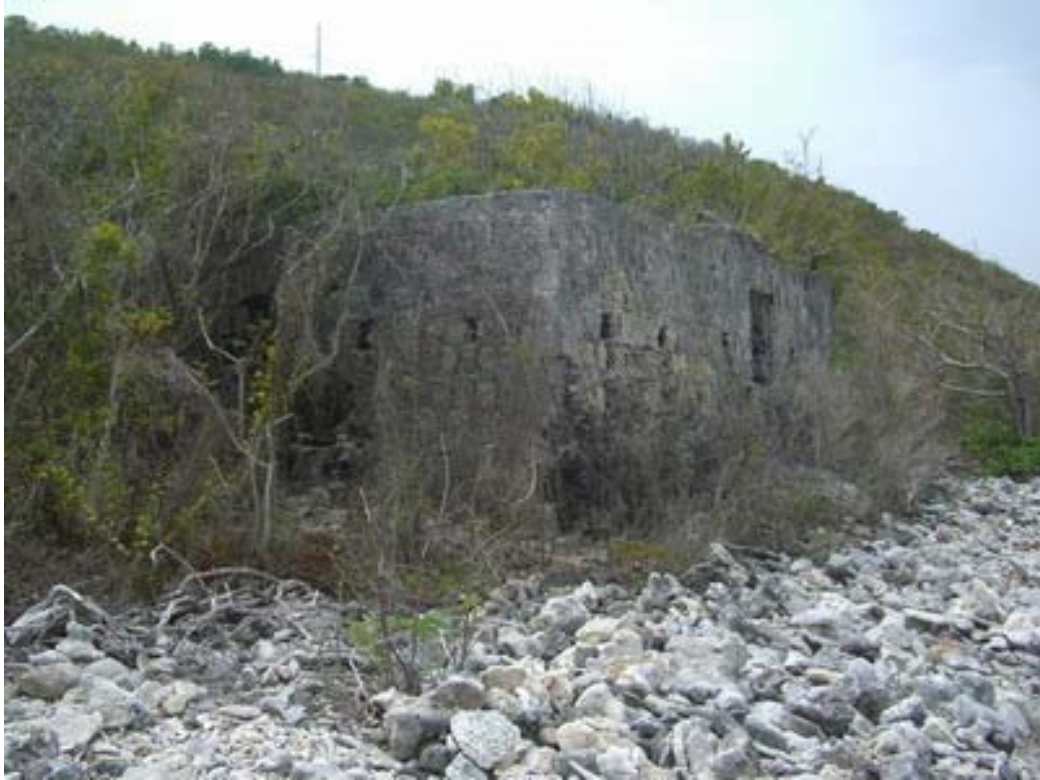
4. The overgrown ruin of the sugar boiling house at Benzies (by the author).
